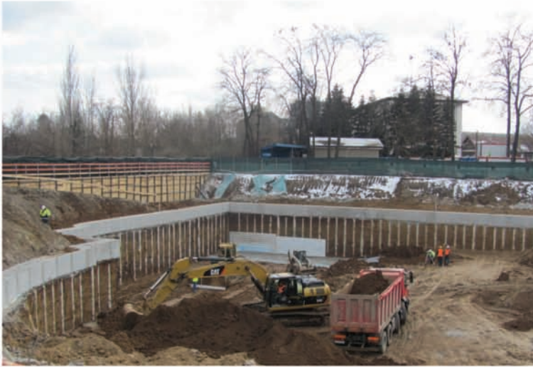
I.G.P.F. OFFICE BUILDING - BUCURESTI
